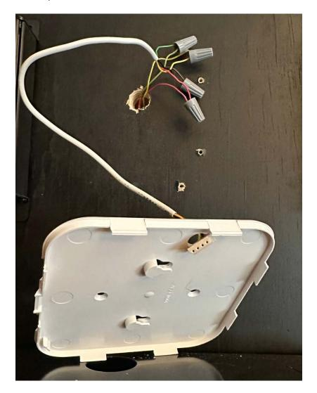
4. Once the wires have been connected and pushed back into the wall, mount the keypad backplate as desired. Use a small level to ensure the plate is level. Use the two fixed mounting holes and not the keyhole positions. Use the supplied anchors if mounting on drywall.
